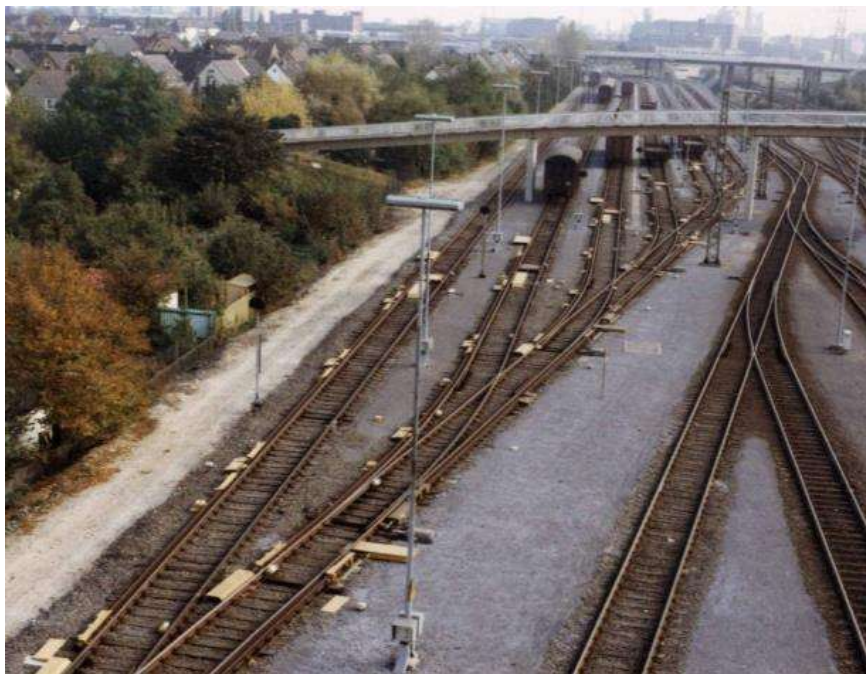
Industrial shunting yard/flat yard (PINPOSITON 400)
